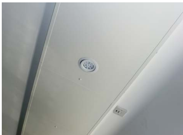
Direct mount panels — plasterboard or solid soffits either around perimeter or in strips
