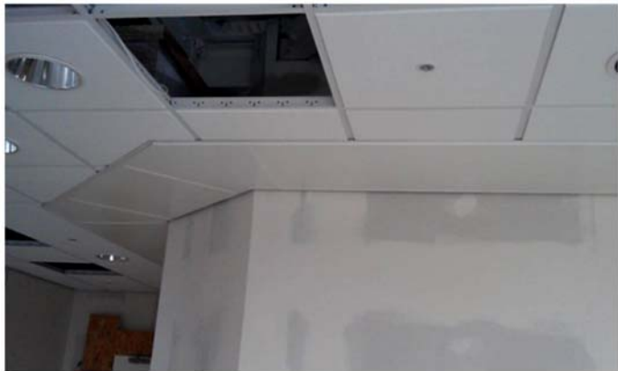
Perimeter panels — high efficiency and comfort leaving the ceiling centre free for other use
