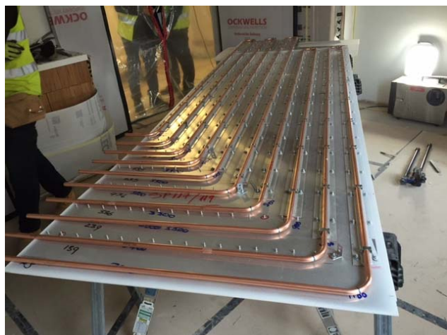
Above example of the back of a radiant cooling panel
