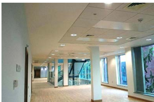
Below an example of ceiling grid mounted panels
