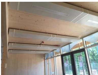
Above: Bespoke perforated panels with lighting integration created for Forrest Educational Centre
