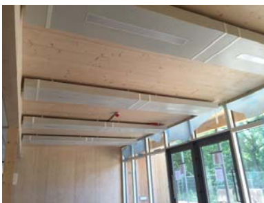
Above: Bespoke perforated panels with lighting integration created for Forrester
