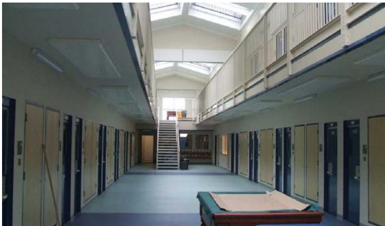
Above, NOMS ceiling mounted panel at HMP Blundeston
