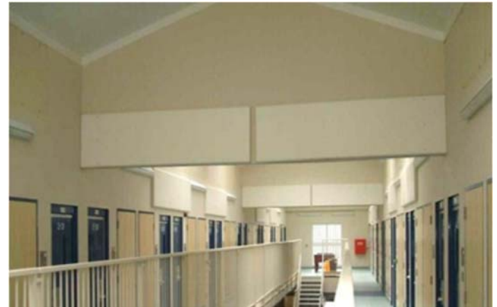
Above NOMS wall mounted panels at HMP Blundeston
