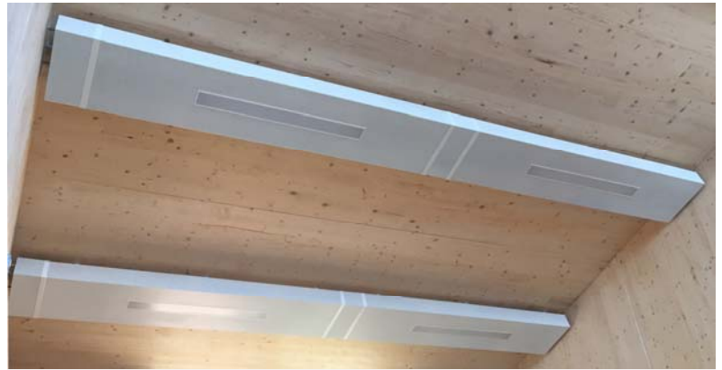
Above Direct mount perforated face panels with integrated lighting at Forest Education Centre, Dibden Purlieu
