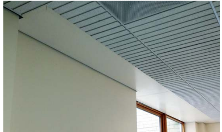
Above Perimeter Panels at Worthing hospital
