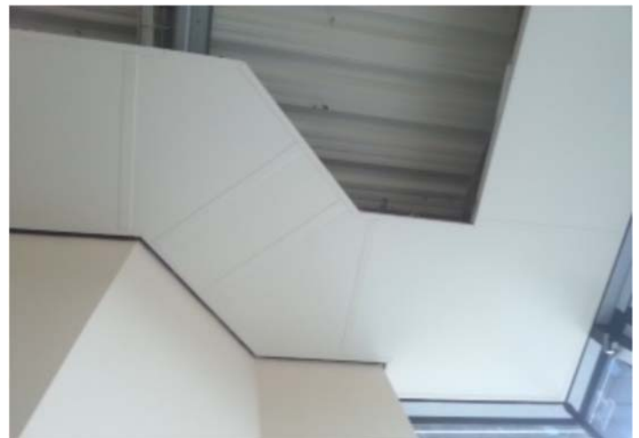
Above Perimeter Panels at Haslingdon Health Centre
