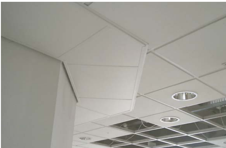
Above Perimeter Panels at Craigavon hospital
