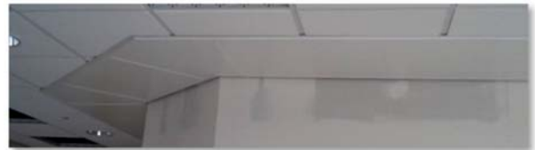
Perimeter panels at Craigavon Hospital, County Armagh
