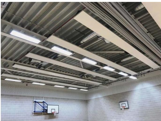
Available in our standard 1.6mm aluminium, 2mm perforated aluminium (for improved acoustic properties) or 2mm steel for areas where an anti-vandal panel is required. Solray FH panels are extremely robust and ideally suited to sports halls where ball games are likely to be played or where other impacts are possible.
