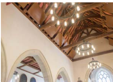
Above, St. Mary's Church in Chalgrove with bespoke colours and mounts with designs in conjunction with CES Lighting &
