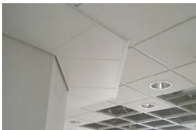
Above: Perimeter Panels at Craigavon hospital following the shape of the room.
