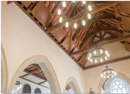
Above and right: Solray radiant panels at St. Mary's Church in Chalgrove using bespoke colours and mounts with designs in conjunction with CES Lighting & Electrical Engineers
